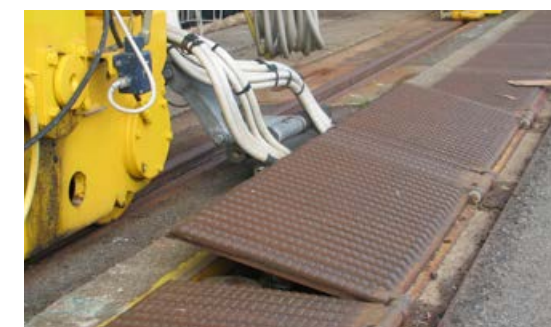
Energy supplied via a busbar of a low-voltage electrical system is also possible.
