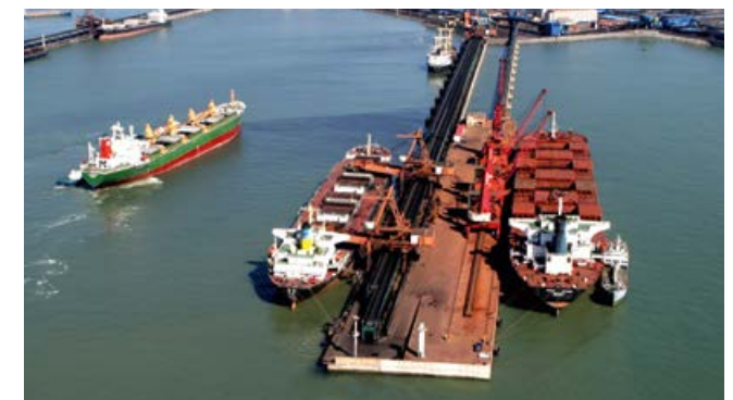
When extending existing quays, portal harbor cranes provide a fast and cost-effective alternative to cranes built for a specific application only.
